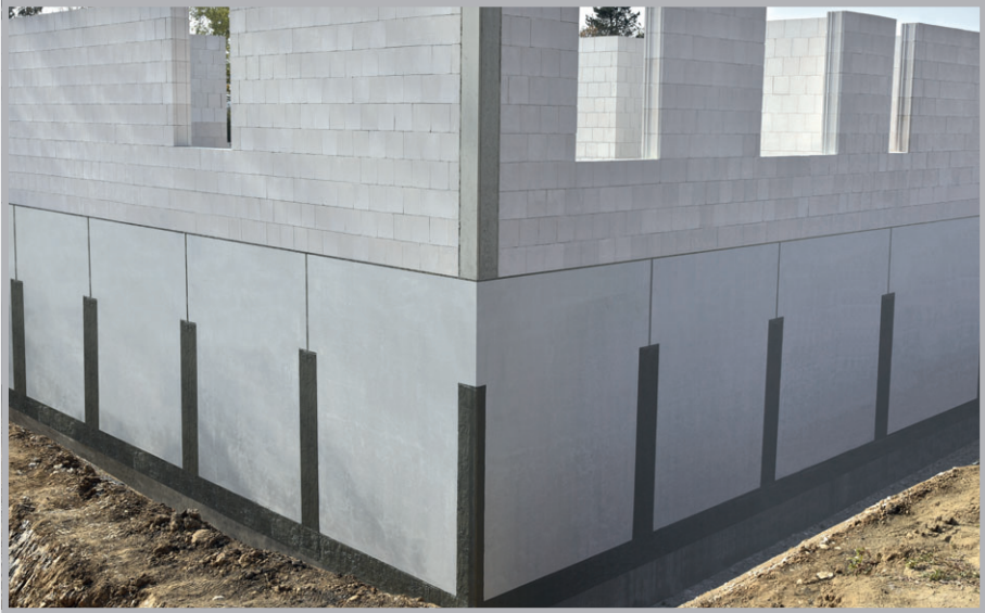
Sealed horizontal and vertical joints
