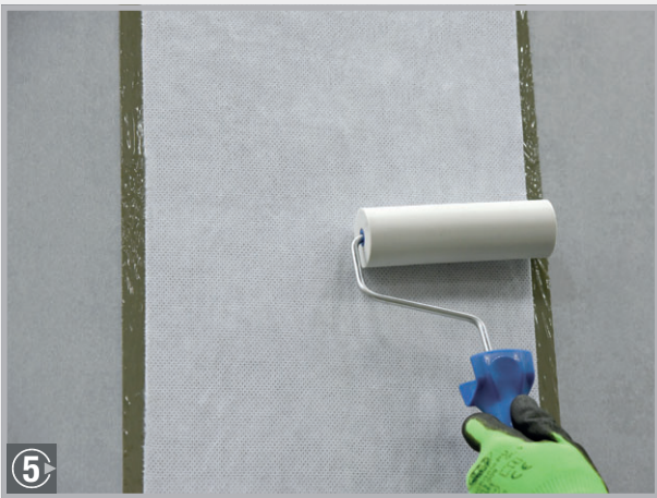
Roll the non-woven into the coating completely with the pressure roller. This step makes it possible to apply the second layer after approximately 2 – 3 hours, depending on the temperature and air humidity.
