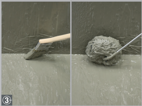
There is a brush and corner roller for the fillet and other areas.
